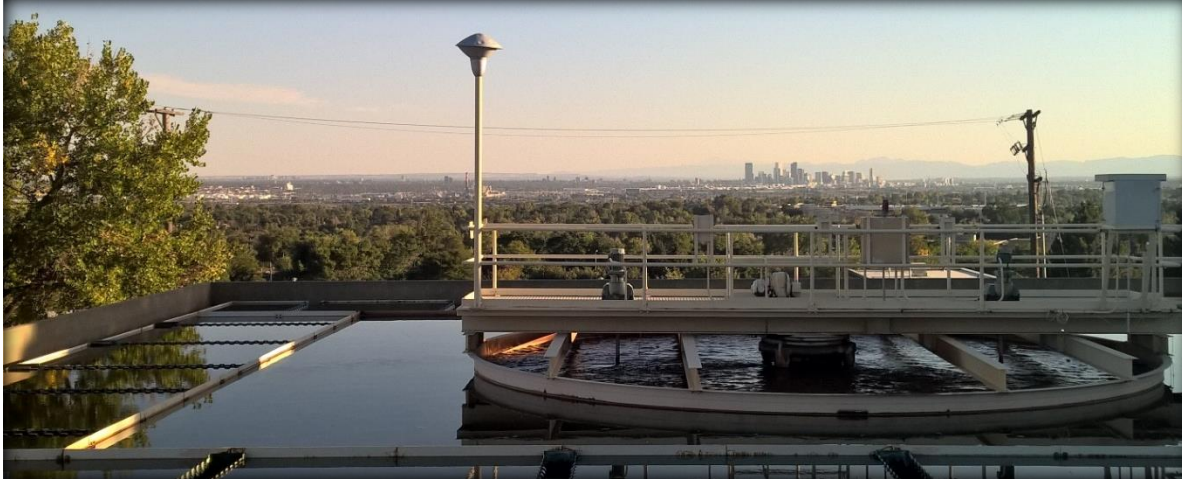
Image 7. Denver Skyline from Clarifiers
