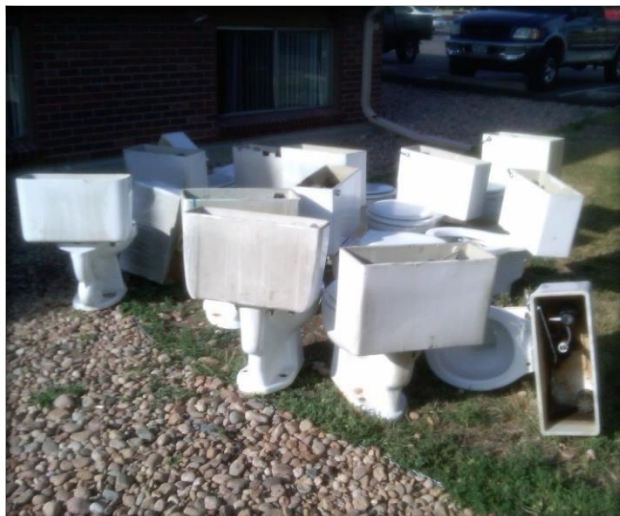
Image 23. Old Toilets Removed from Multifamily Building
