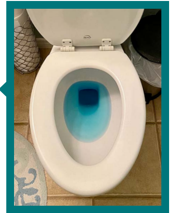
Visible color seeping into the bowl (pictured here) would indicate a leaky toilet.
