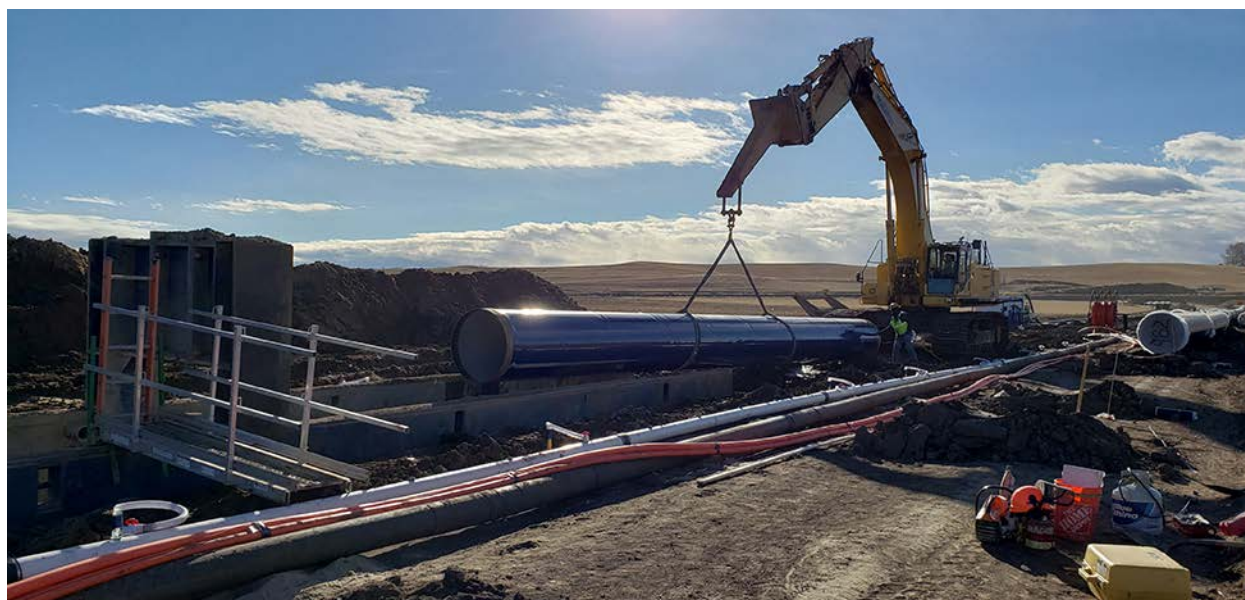
Image 15. Construction of Thornton Water Pipeline
