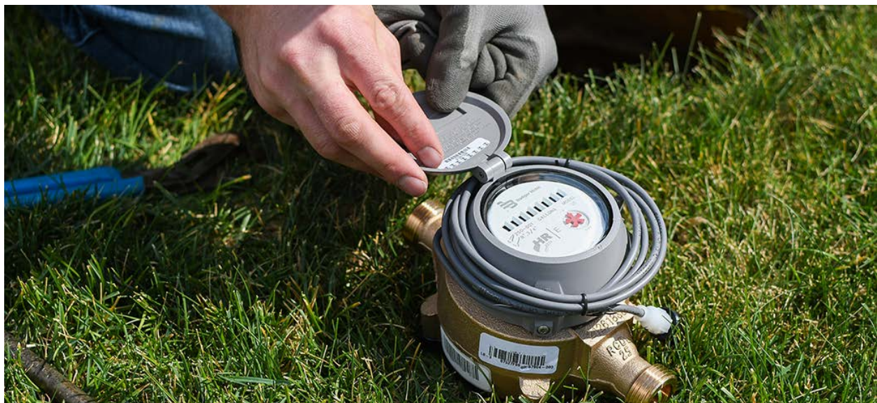
Image 19. Thornton Water employee installing a new water meter
