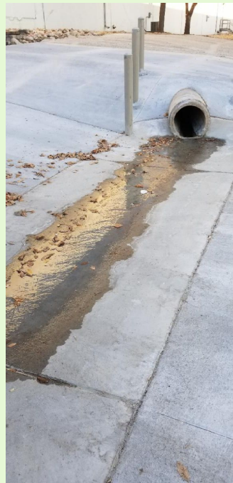
Groundwater on pavement coming out of a drainage culvert.
